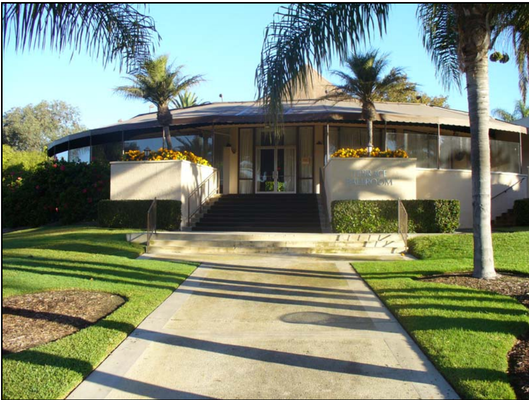
Figure 4. 1960s Terrace Ballroom slated for demolition
